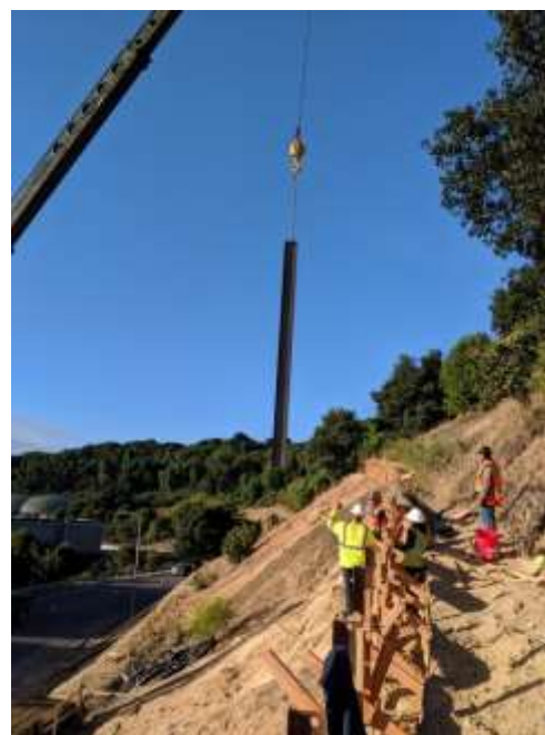
Retaining wall construction
