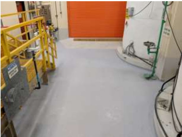
New coating in the sodium bisulfite storage room
