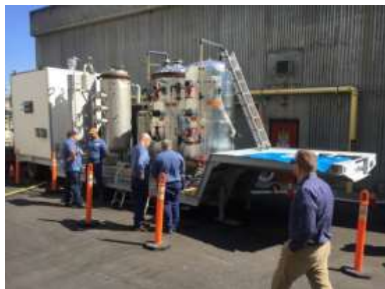
CMSA staff constructing upgrades to the pilot study equipment
