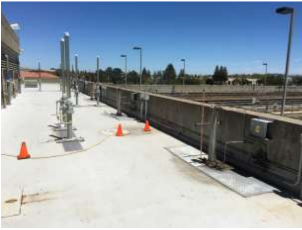
Old hydraulically-operated primary clarifier gate actuator systems (left) and new electric actuator(right)
