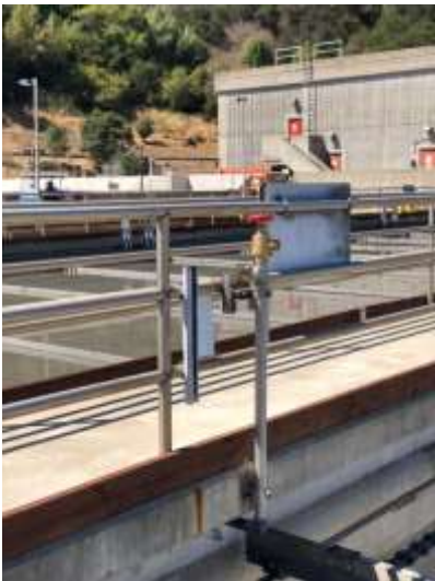
Piping installed under the decking for UV protection
