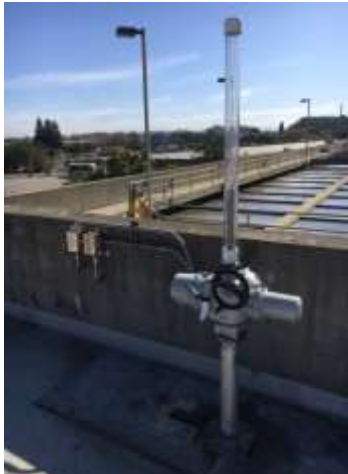
Old hydraulically-operated primary clarifier gate actuator systems (left) and new electric actuator(right)
