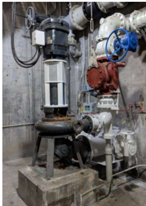
Direct-coupled pump with enclosed rotating equipment
