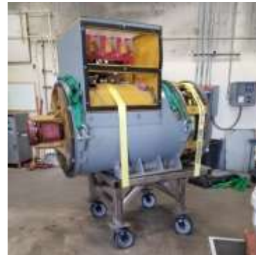
Generator prepared for offsite repairs
